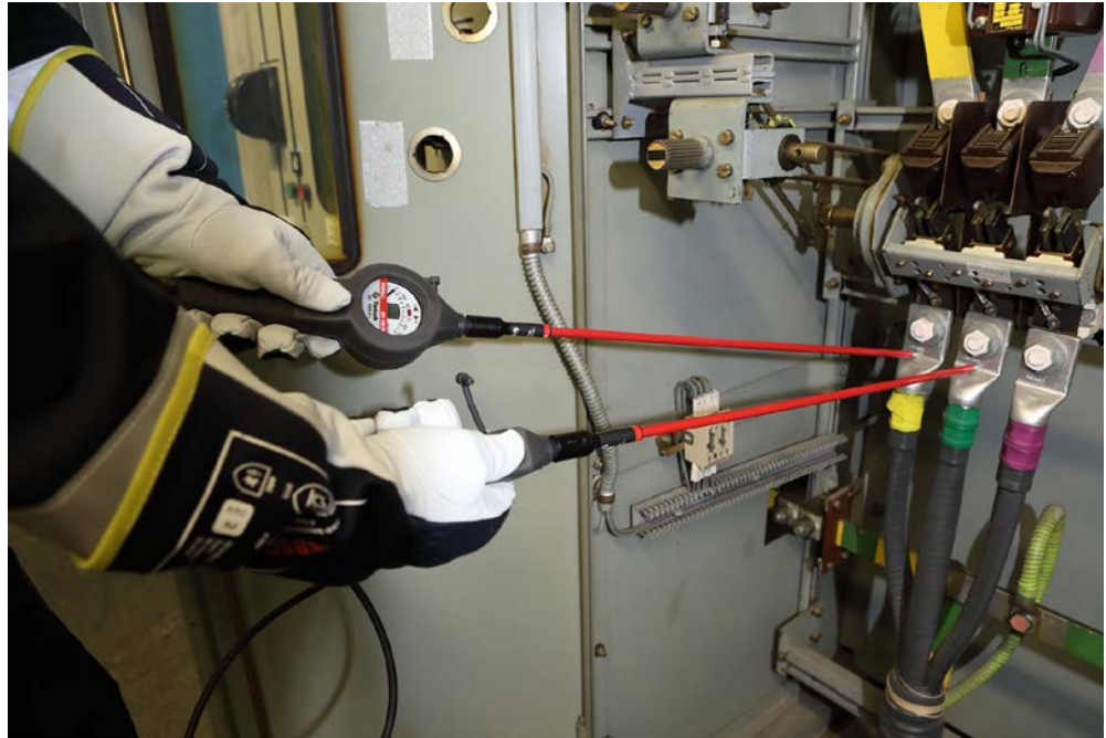
Fig. A 5-22 Determining a voltage-free state
