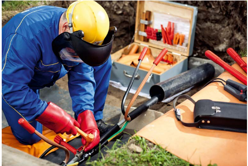
Fig. A 5-6 Working on a cable sleeve
